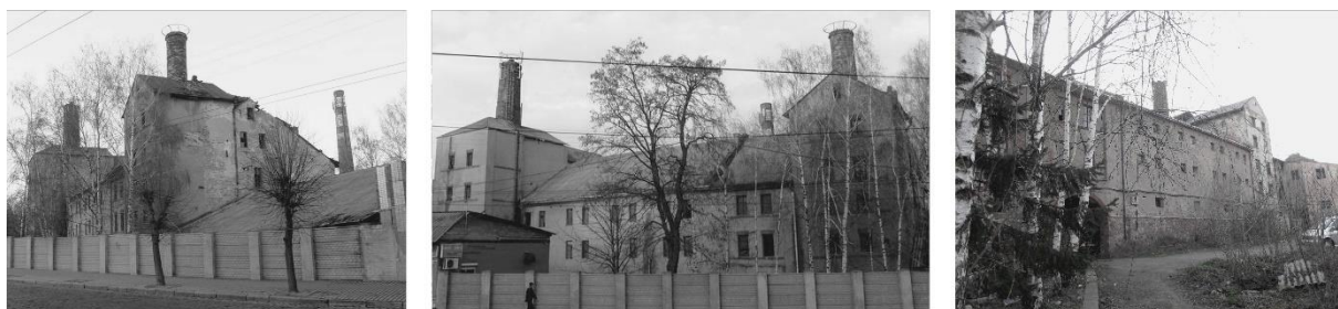
Fig. 3. The current condition of the brewery
